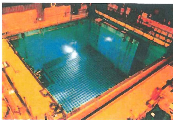
Figure 4: Spent fuel storage pool (Source: Union of Concerned Scientists)
